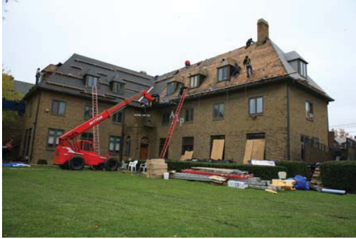
Roof under construction: Phi Kappa is finally keeping dry!
